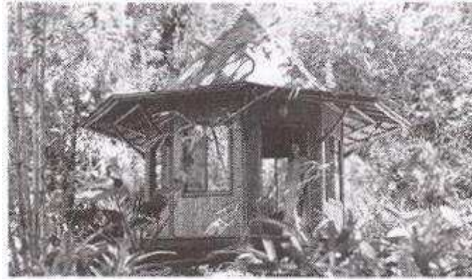
Fig. 8: A Small structure created using locally available material-saves cost.
