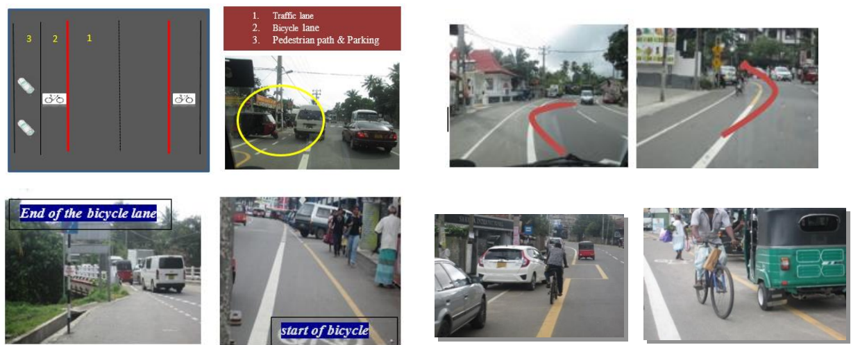
Fig. 8: Blocked the bicycle lane by other vehicles: Piliyandala Bicycle lane
