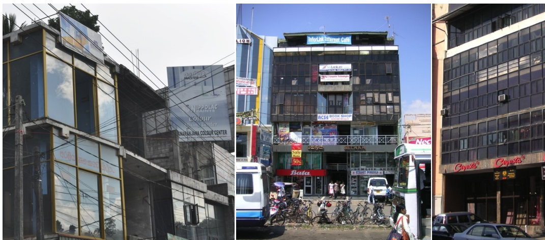
Fig 2: Contemporary, urban, commercial vernacular Source: Authors
