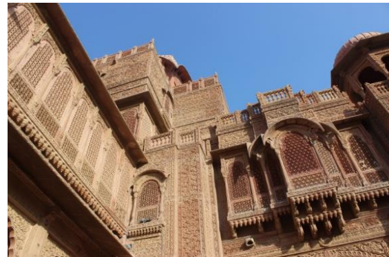
Figure 9: Thick walls in sandstone provides heavy thermal mass
