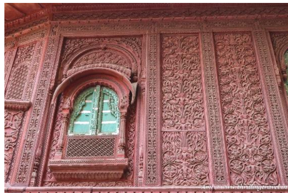
Figure 12: Textured surface reduces solar absorption
