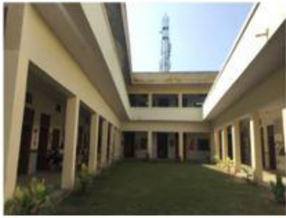
Figure 17: Central courtyard as the sole spill-out space Source: author
