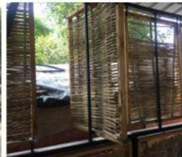
Figure 31: Windows made of thatch and bamboo Source: author
