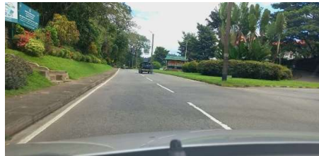
Figure 33: Soft Road shoulders and Road Islands in Peradeniya Old Road. Source: author
