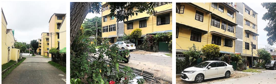
Figure 4.28: Wide internal streets forming spacious pedestrian space
