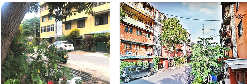
Figure 4.32; Spaciousness in layout design clean atmosphere making residents appeal onto the living setting
