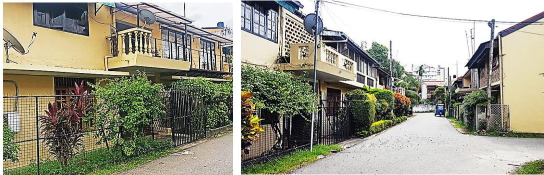
Figure 4.34; Additions and alterations including fencing, fulfilling the requirements of individual identity yet does not harm the overall character.
