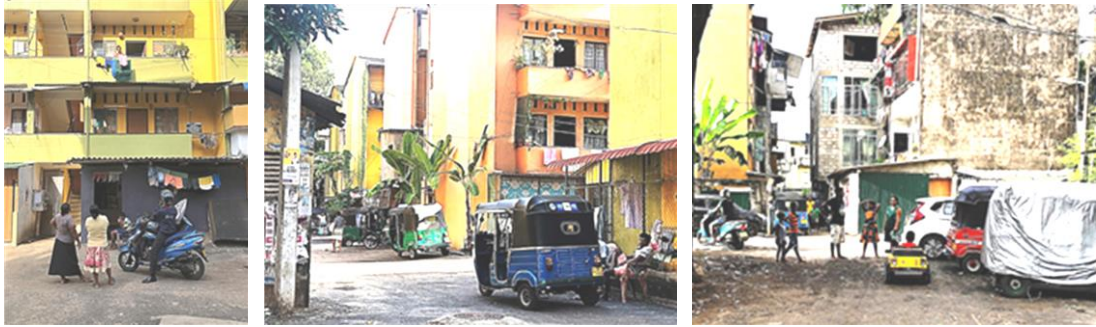
Figure 4.17: Internal roads and extended open areas create interactive communal spaces within the neighbourhood; for children to play and adults to hang-around
