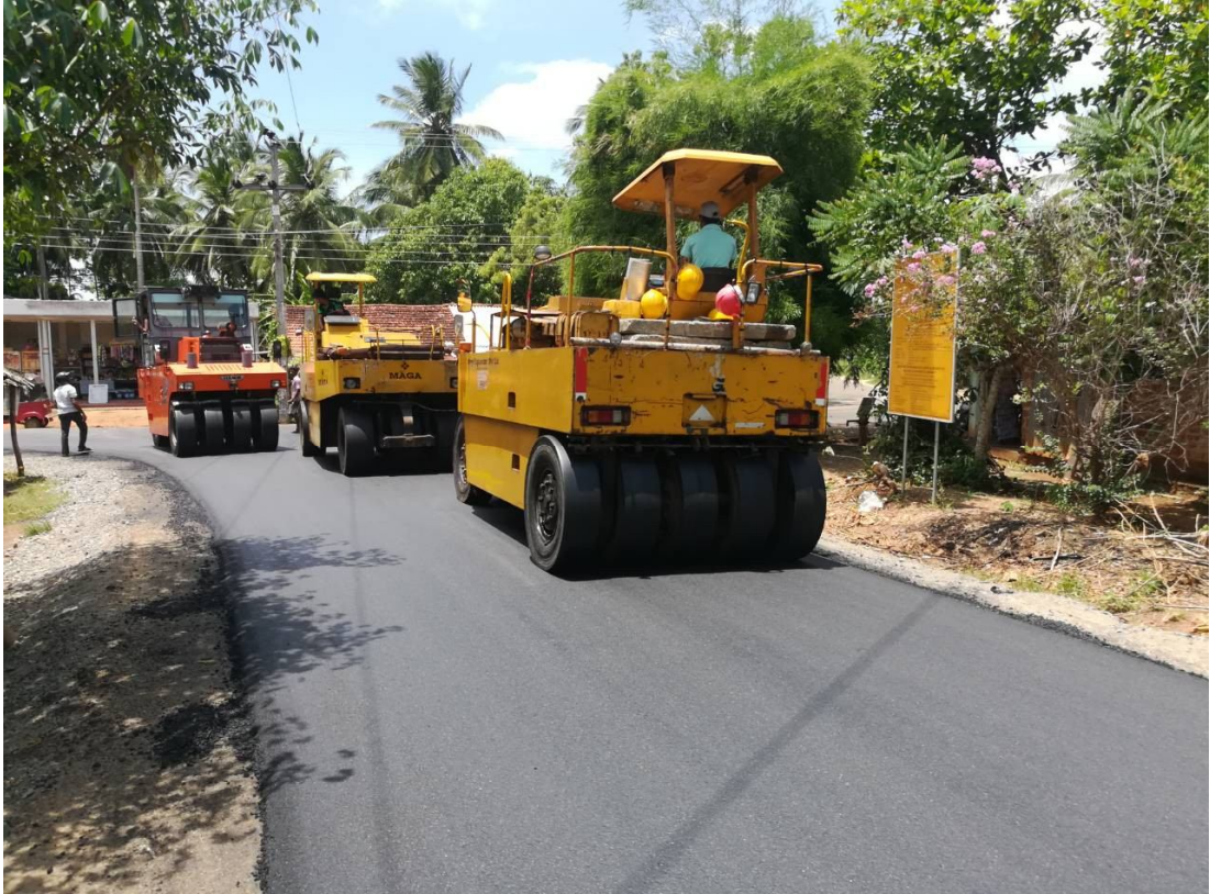
Figure 3-2 Compaction of HMA (AP4 Project)
