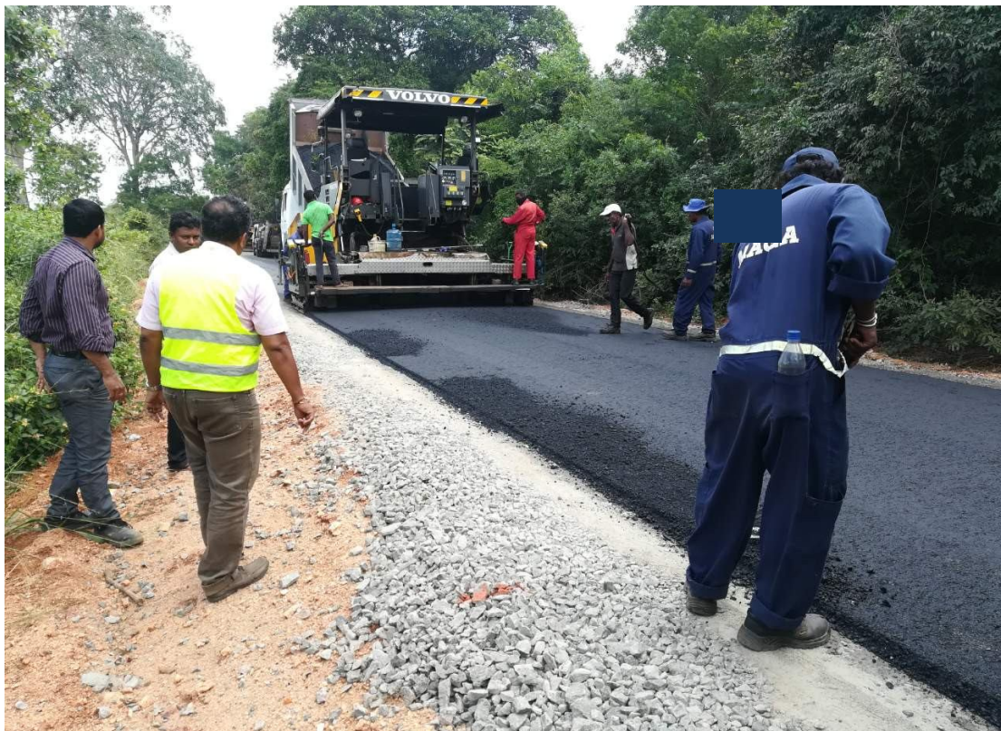
Figure 3-1 Laying of HMA (AP4 Project)
