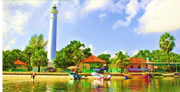
Figure 37: Aesthetic design elements at the Light House Park Source: Author
