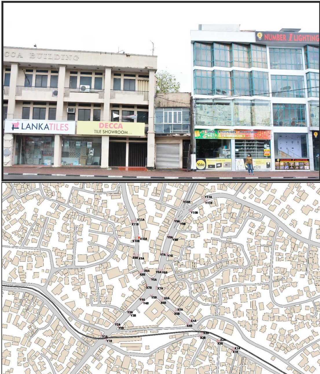
Figure 71: Photograph and Location of surveyed point X10A; Source: Author
