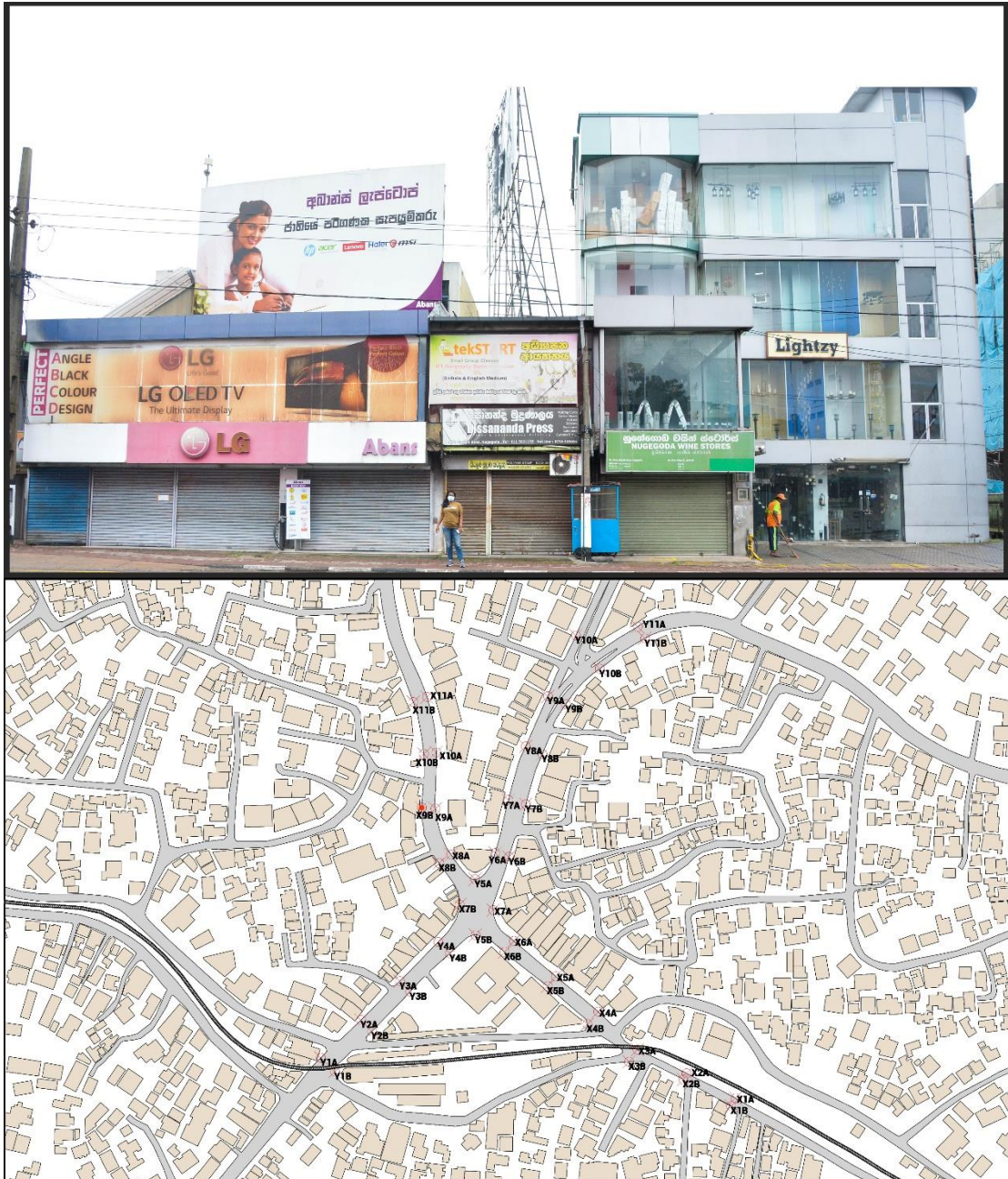
Figure 69: Photograph and Location of surveyed point X9B; Source: Author
