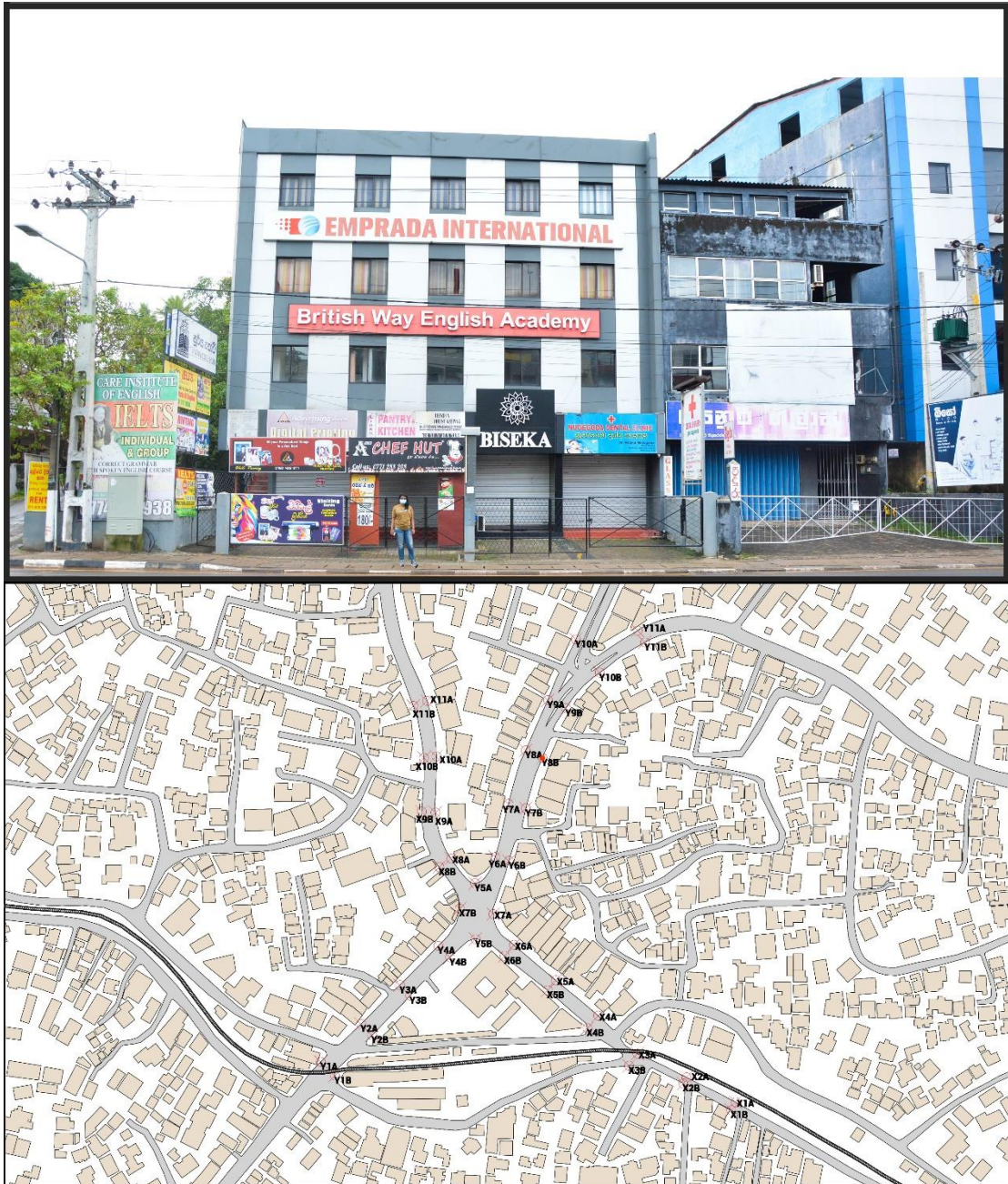
Figure 109: Photograph and Location of surveyed point Y8B; Source: Author
