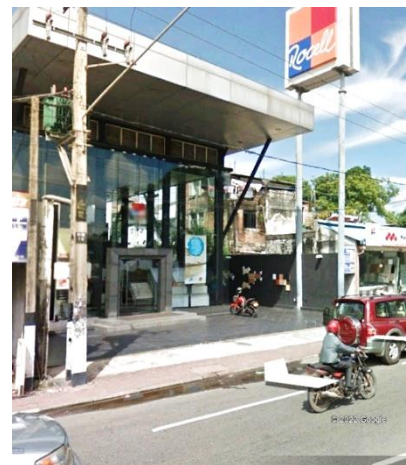
Figure 42: Rocell building maintaining building set back [Photograph] Source: By Author
