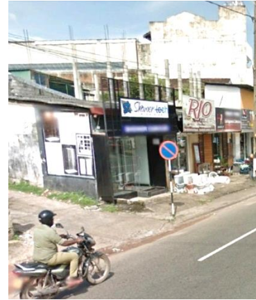
Figure 43: Small scale shops without proper set back [Photograph] Source: By Author
