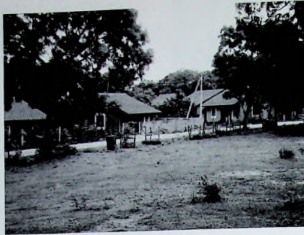
Fig. 11 Housing Village in Hambantota District is built in an appropriate scale though its composition fails to provide for facilitating of small scale communal spaces.
