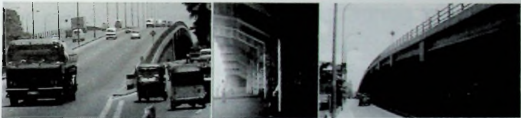
Fig. Form of the flyover is easily graspable, the elements consisting in the form
