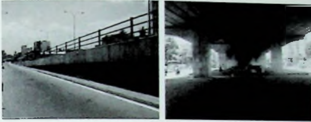
Solid barriers and the voids for visual contacts through the supportive structure of the flyover.
