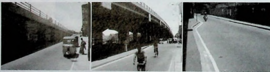
Fig. Directionality of the flyover reduces the robustness; the solid ramp which inclines, the overhead edge runs, the narrow paths at the both side of the flyover.
