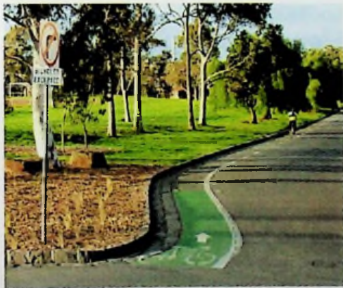
Figure 2.13: Road marking and Colour surface demarcated for cycle users
