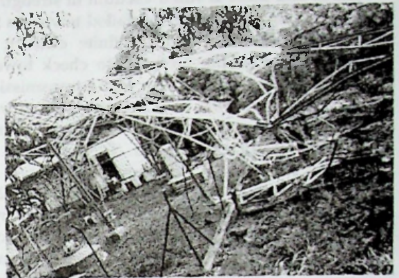
Fig 2 Mihinthale 70m antenna tower collapse
