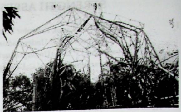
Fig 2 Mihinthale 70m antenna tower collapse
