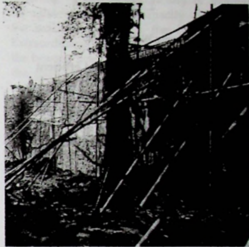
Figure 04: Neighbours Side of Retaining Wall - Type 2
