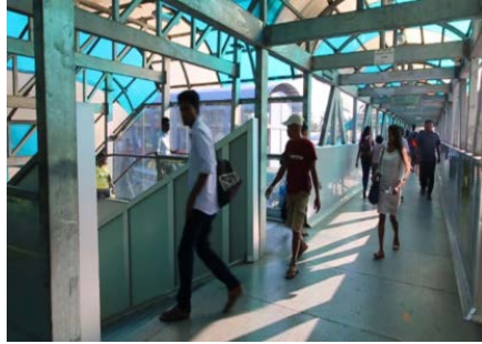
Figure A.2: Panadura Pedestrian Bridge - L2
