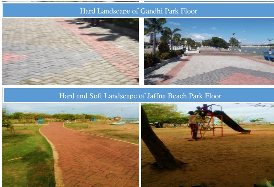
Figure 32: Hard Landscape of Gandhi Park Floor and Hard with Soft Landscape of Jaffna Beach Park Floor Source: Author
