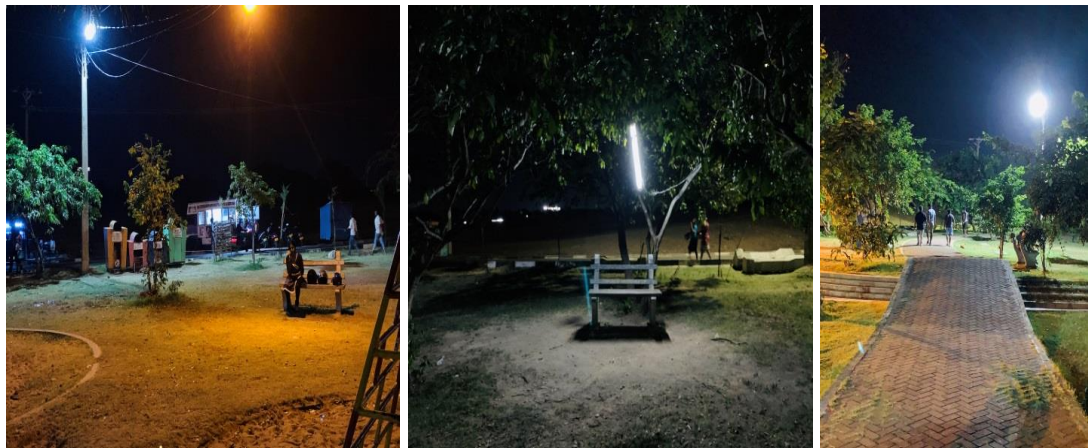
Figure 41: Illuminate Light Arrangement inside the Jaffna Beach Park Source: Author
