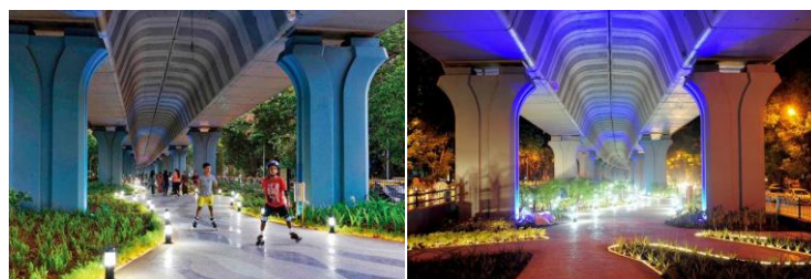
Fig.04 : Under flyover garden in Mumbai, Source:Internet
