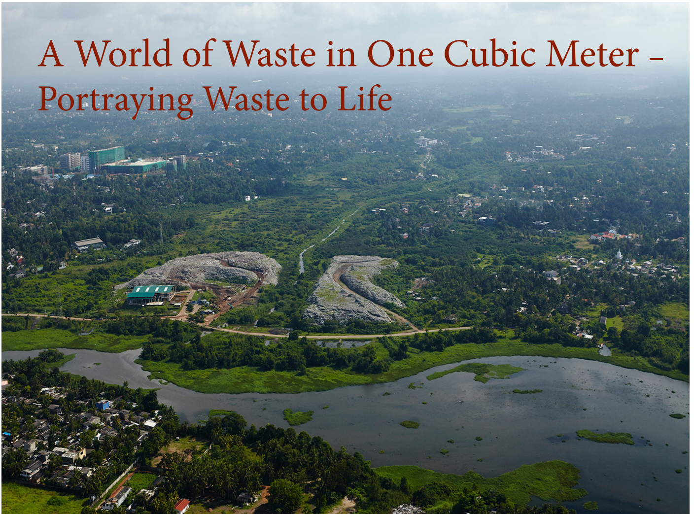
Figure 1: Aerial View of Karadiyana solid waste site – University of Moratuwa is in the background
