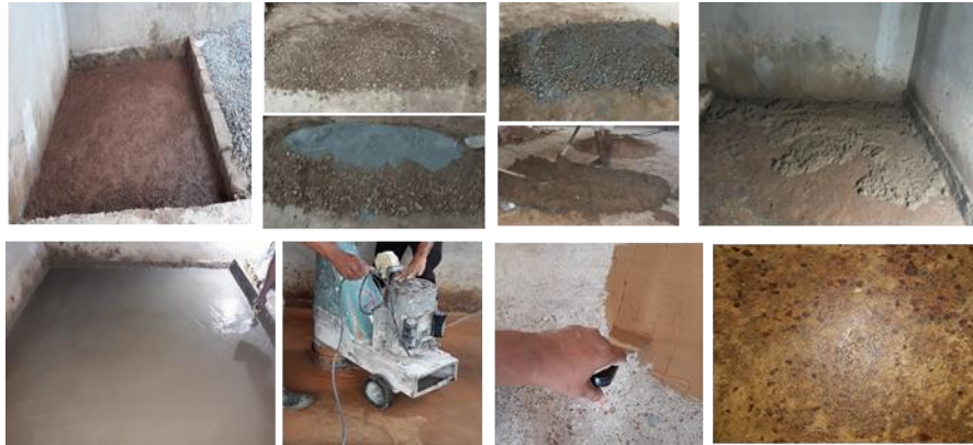
Figure1: Step of soil floor construction
