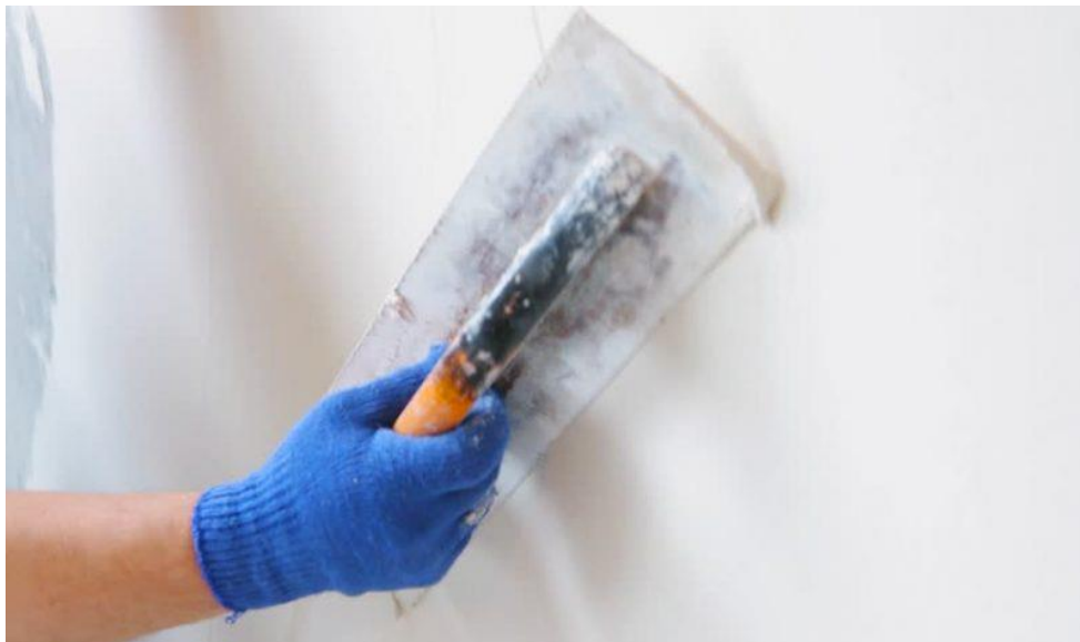
Figure 2.1: Joint compound application using a putty knife
