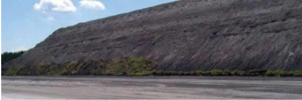
Figure 1-3: Dry disposal method of fly ash
