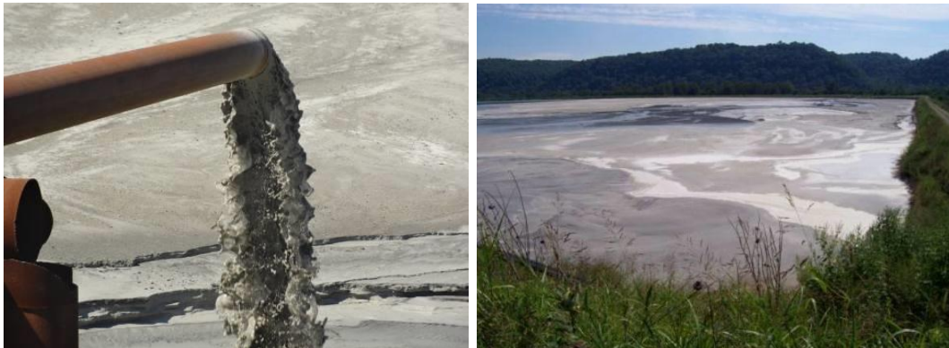
Figure 1-2: Wet disposal method of fly ash
