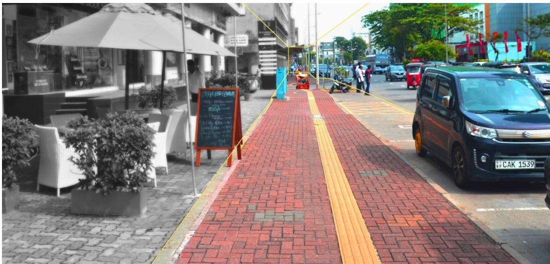
Figure 6: On street Parking, Bagatale road
