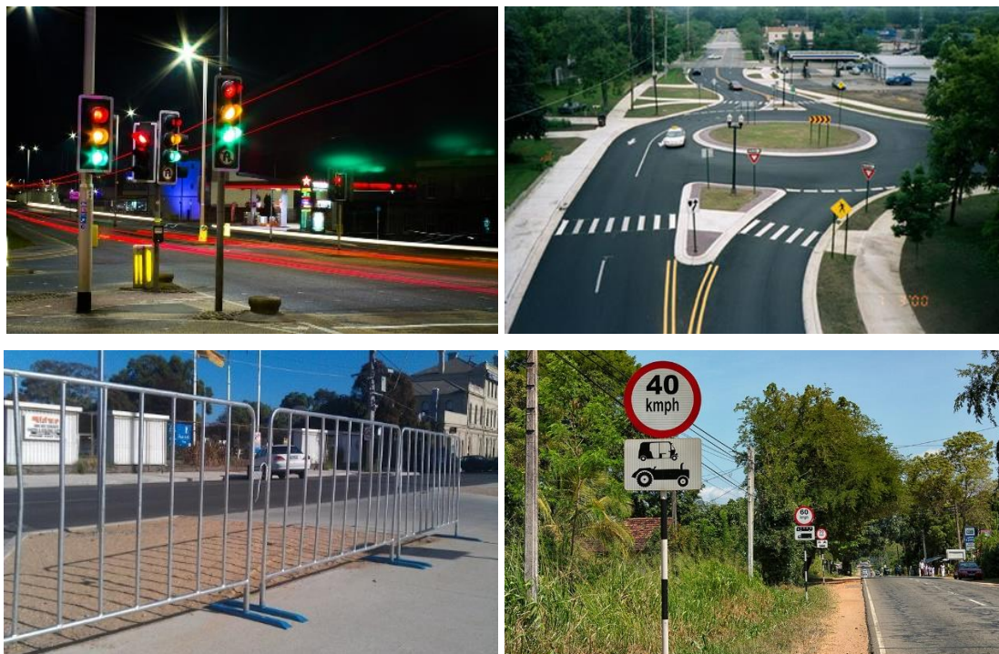
Figure 9: Traffic related roadway installations
