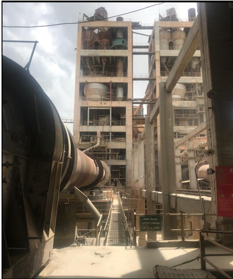
Figure 4.1: Cyclone tower and kiln at INSEE cement plant
