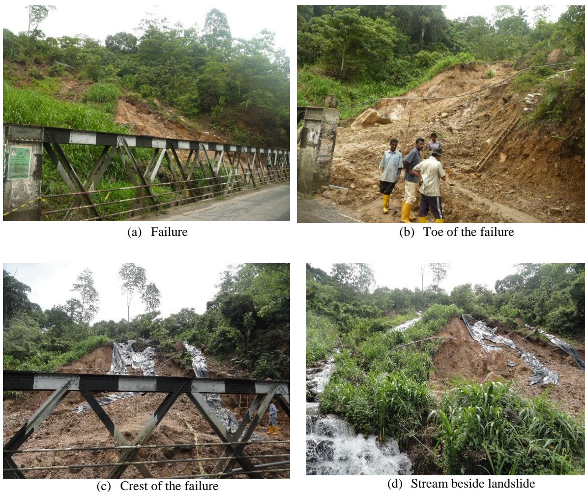
Figure 3.2 : Landslide on June 2014 ( National Building Research Organisation, 2014 )
