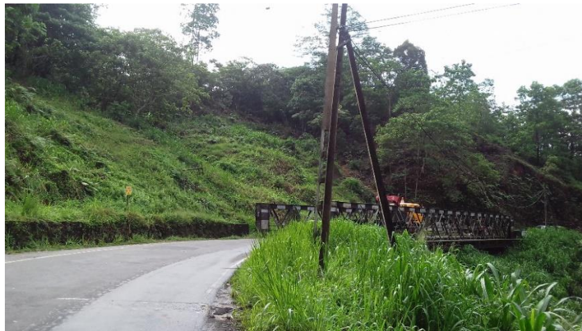
Figure 3.3 : Ginigathhena Landslide Body
