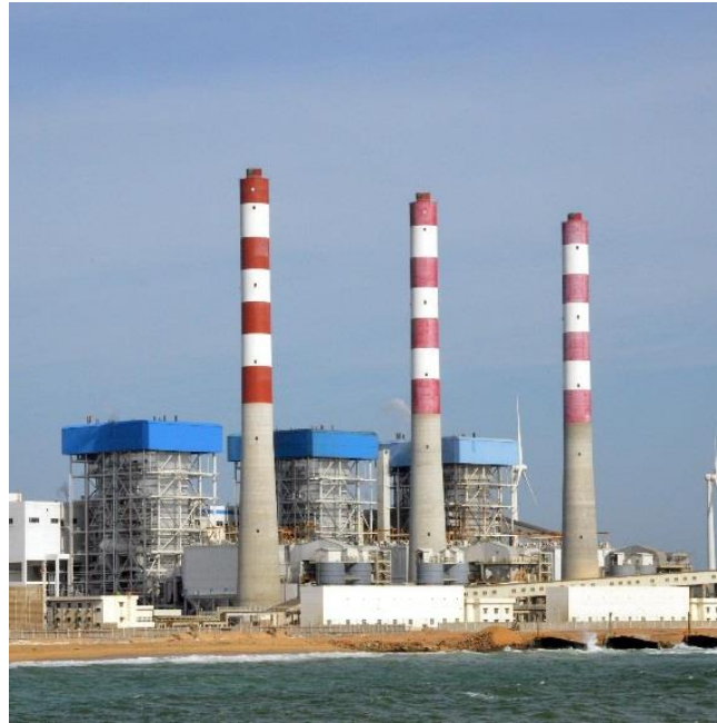
Figure 1.2: Lakvijaya thermal power plant located in Norochholei, Sri Lanka (Source: web)
