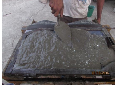
(b) Spreading the mix on the vibrating table
