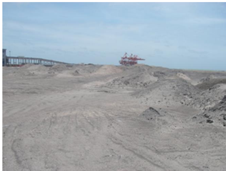
Figure 1.3: Coal fly ash is being dumped in the open yard at Lakvijaya power plant
