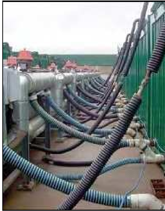
Figure.2.57: Each static container is attached to a central air system using flexible hoses[17]
