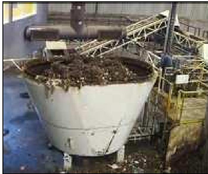
Figure.2.34: Vertical mixer used at a composting facility [17]
