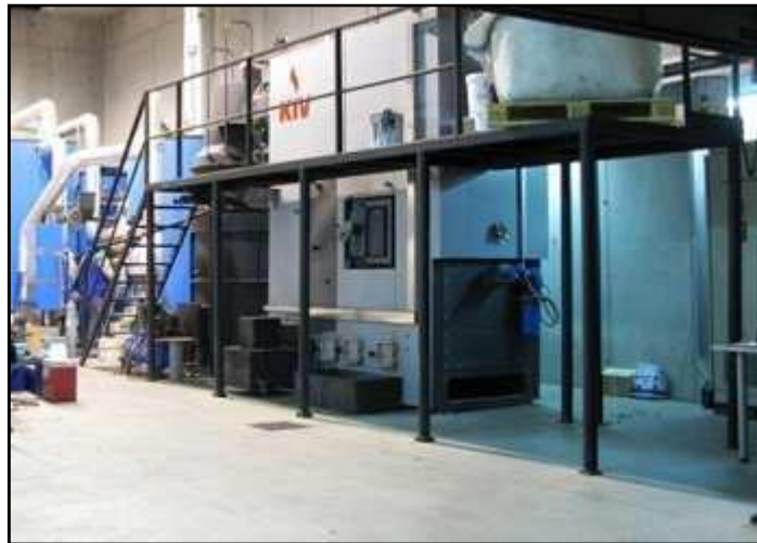
Figure.2.8: Pilot scale W-t-E gasification plant during experiments and investigations [3]
