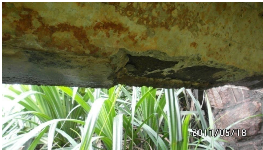
Figure 3-7: Initial stage of spalling due to corrosion of reinforcement
