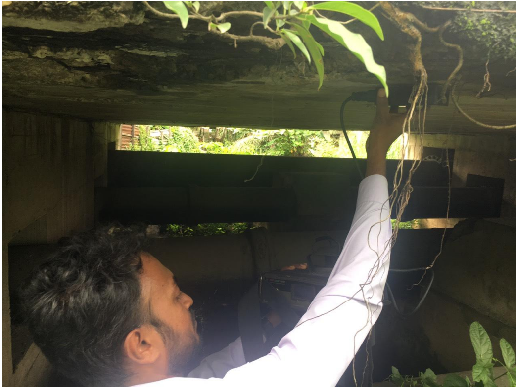
Figure 3-26 : Taking readings with cover meter on an old bridge deck
