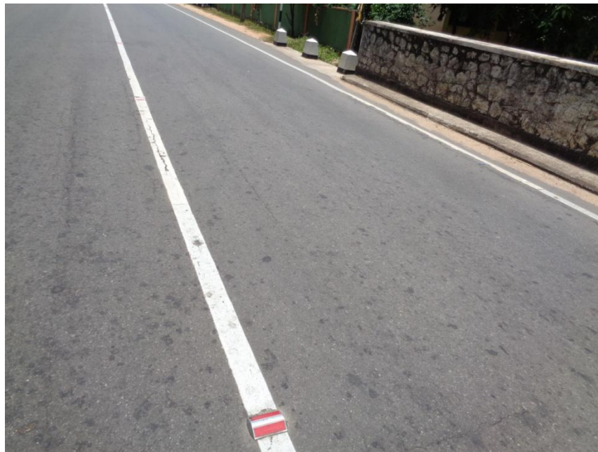
Figure 3-12: Relative vertical displacement between beams due to malfunctioning of diaphragm
