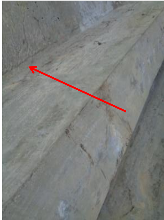
1 - Shear crack
