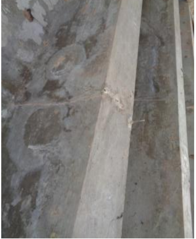
2- flexural crack
