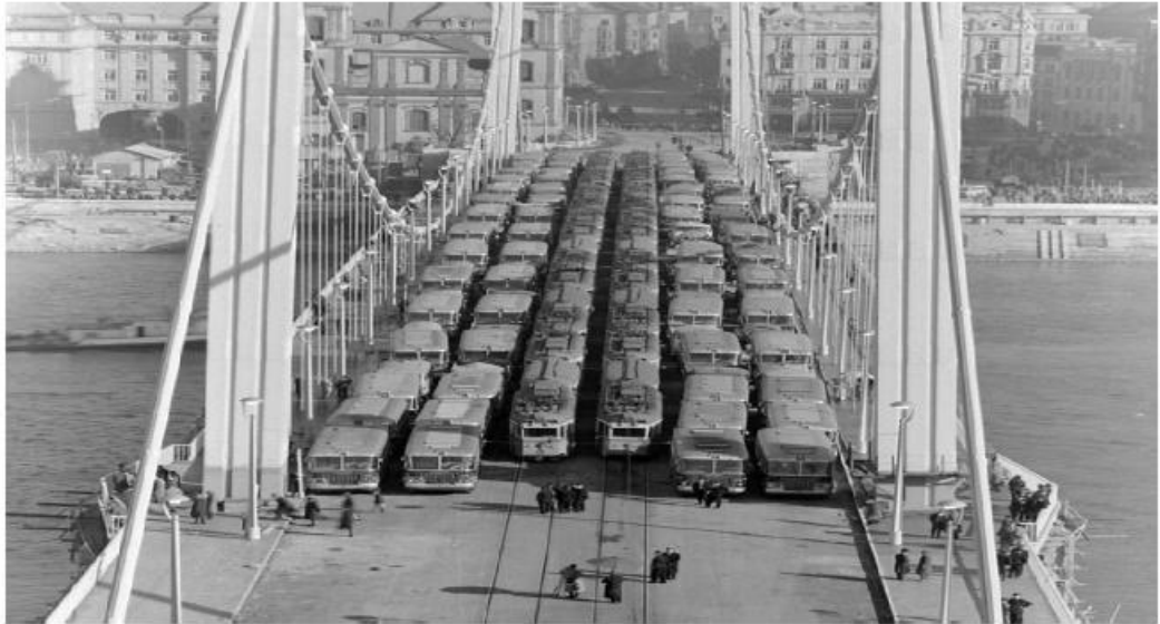
Figure 2-13: Proof load test on New Elizabeth Bridge in 1964 [17]
