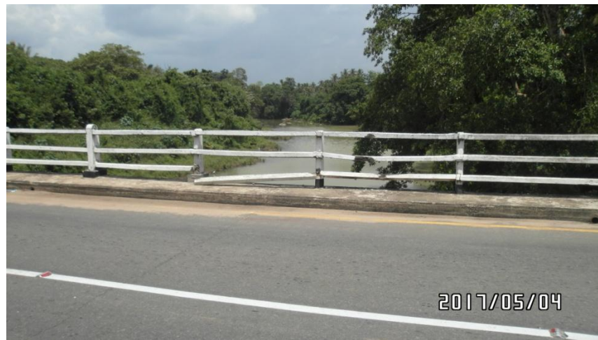
Figure 3-17: Damaged handrail
