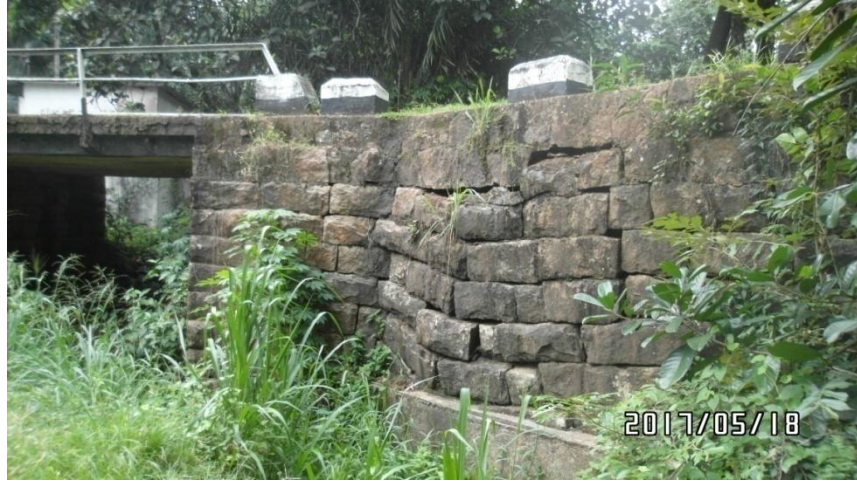
Figure 3-19: Lateral movement of dressed stone wingwall
