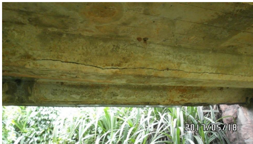
Figure 3-7: Initial stage of spalling due to corrosion of reinforcement
