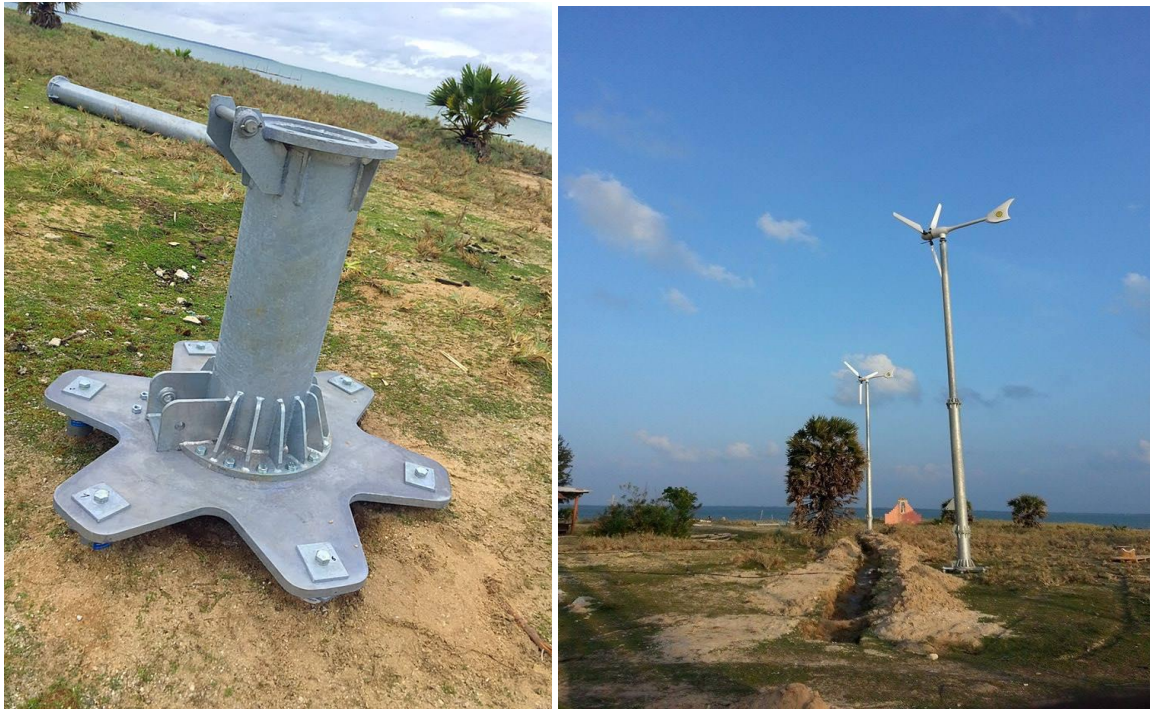
Figure 5.7: Base of a wind turbine and two wind turbines operating at the site.
