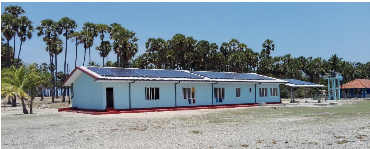
Figure 6.1: the powerhouse of the Hybrid distribution system at the site
