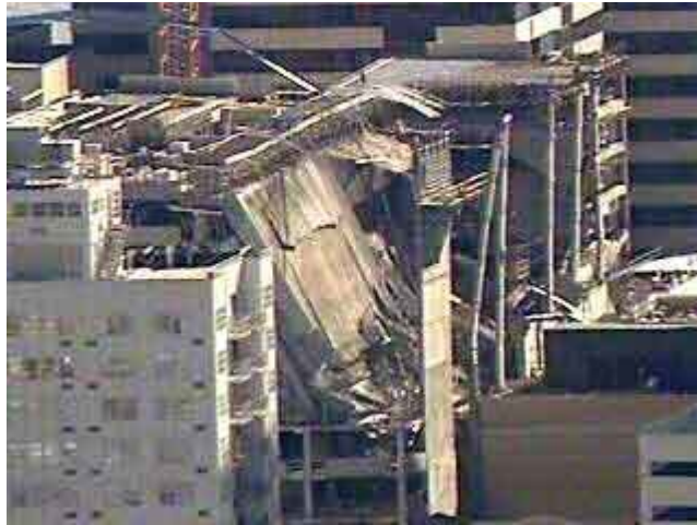
Figure 2.3- Flat slab failure an earthquake (Tropicana Casino Parking Garage)
