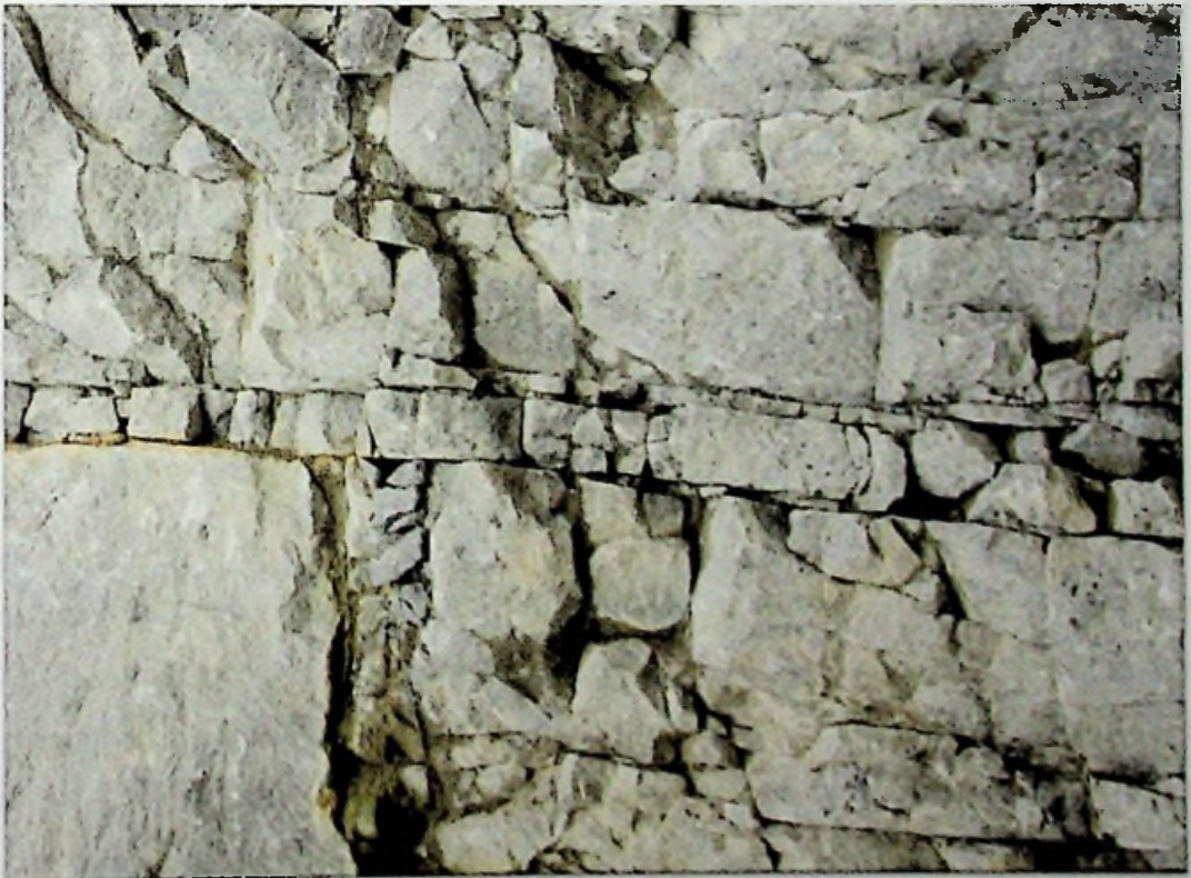
Figure 3.3 :Fractures and Joints
