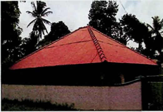
Figure 2.10: Four Pitch painted asbestos roof
