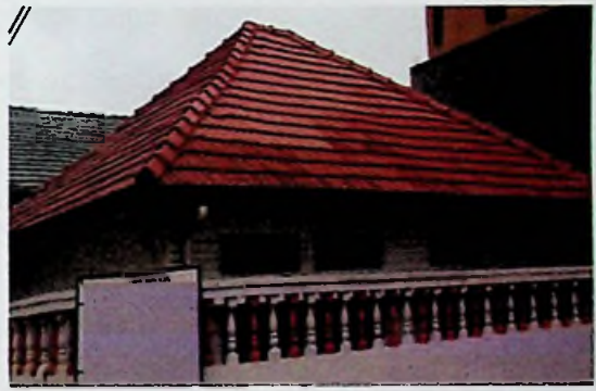
Figure 2.11: Four Pitch calicut tile roof
