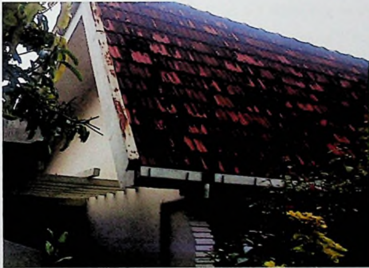
Figure 2.3: Pitch Calicut tile roof
