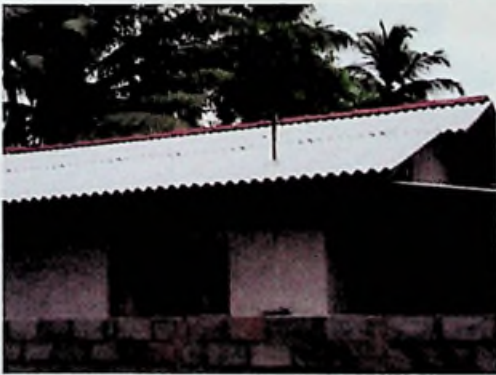
Figure 2.7: New asbestos sheet roof
