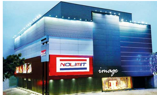
Figure 5.10: Exterior view Source: http://www.nolimit.lk
