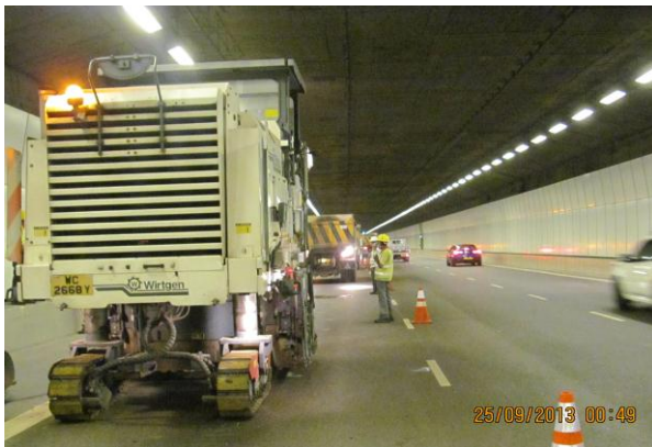
Work carried out within a single lane closure
