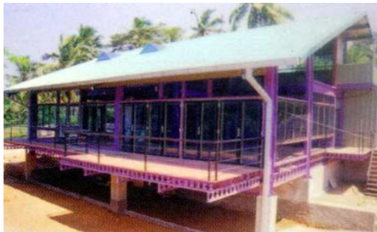
Figure 4-20: Fully factory produced and site assembled steel house at Bolgoda, ABS (pvt) ltd- Kaduwela.
