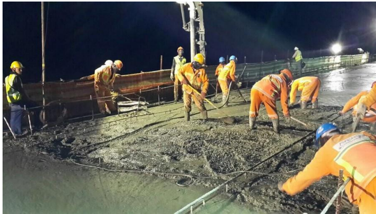
Figure 2-7: Usage of ready mix concrete (Source: stallionreadymix.co.za)
