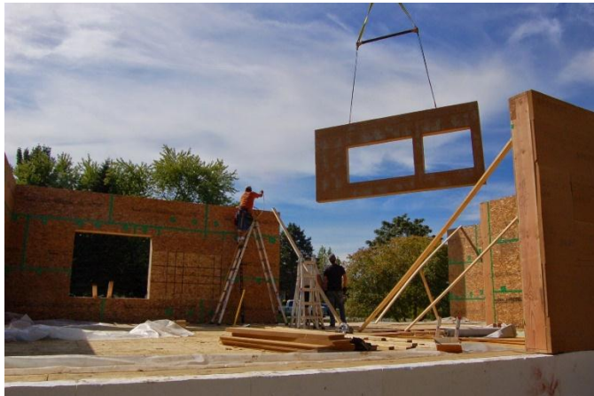
Figure 2-10: Assembling of prefabricated wall panel (Source: greenbuildingadvisor.com)
