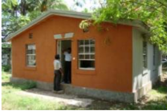
Figure 4-17: External view of a wall coloured model house, NHDA - Maligawatha
