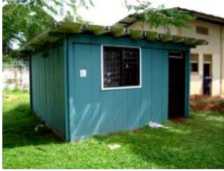
Figure 4-40: Prototype house done by the NERD Center using prefab cement panels
