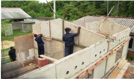
Figure 4-12: Assembling of the prefabricated model house, NERD center - Ekala.
