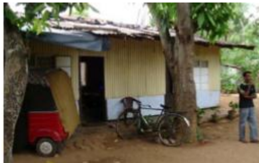
Figure 4-2: Front view of RVDB workers' houses At Udawalawe
