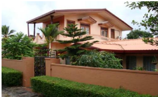
Figure 4-32: A twin type house at Rukmalagama converted to a two-story one while the original walls remain same.
