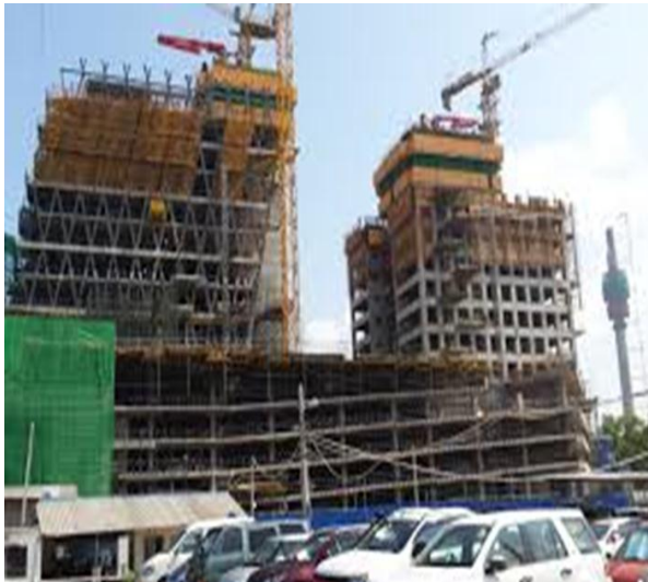
Figure 2-9: Beginning stage of Altair twin tower
