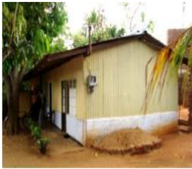
Figure 4-1: External view of RVDB workers' house at Udawalawe
