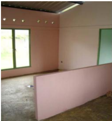
Figure 4-25: Three Inch thick partition wall, model house - NERD center.
