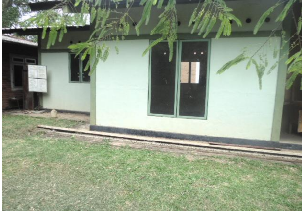
Figure 4-14: External view of NERD model house after finishing.
