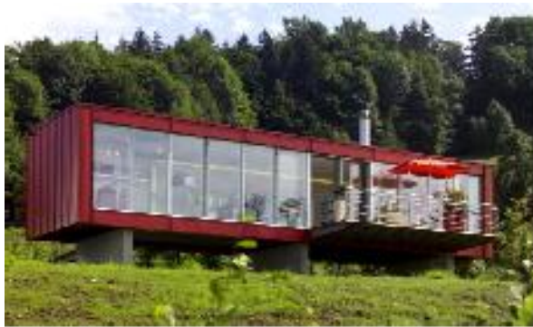
Figure 2-11: Fully factory produced residential unit at a rural area
