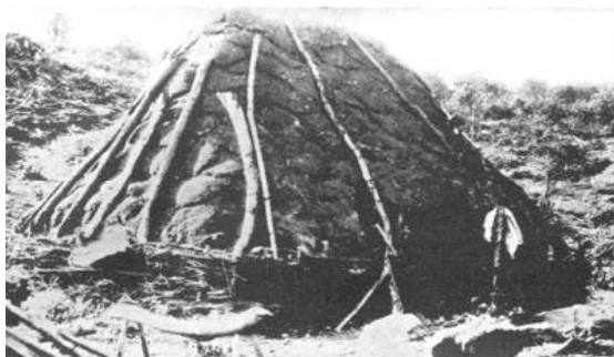
Figure 2-1: An ancient Iron–Age hut made of clay and wood (Source: www.solohq.solopassion.com )
