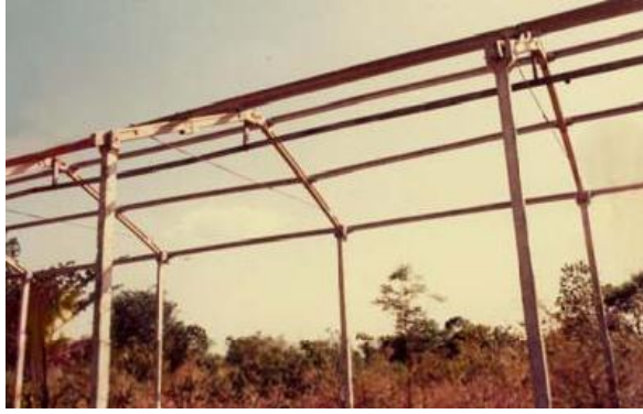
Figure 4-4: Frame structure of RVDB house at Morakatiya
