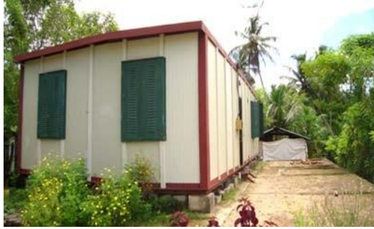
Figure 4-11: Placement of the kit-house on the foundation of destroyed house.
