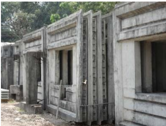
Figure 4-19: Prefabricated wall panels produced by the ICC – Piliyandala
