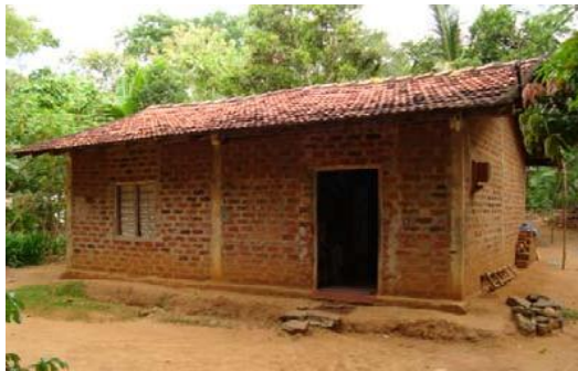
Figure 4-5: Only frame structure is prefabricated RVDB house at Morakatiya.
