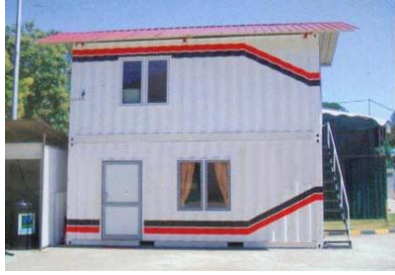
Figure 4-21: A residential container conversion, Mclerence Logistics Pvt. Ltd.- Walissara.
