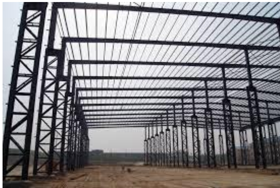
Figure 2-8 : Steel structure for long spans (Source: alibaba.com)
