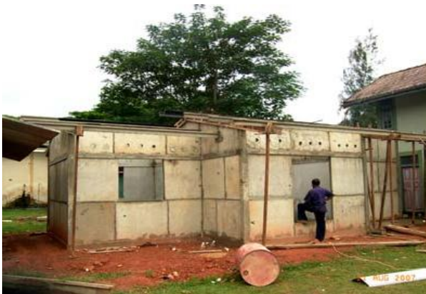
Figure 4-13: External view of the NERD model house before finishing.
