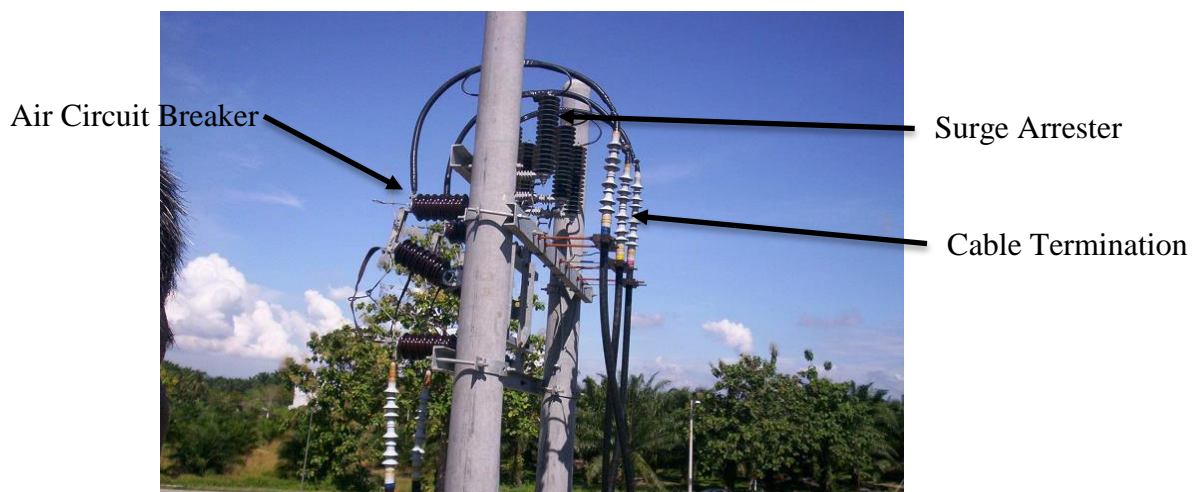
Figure 3-5: Installation of SA where ACB placed in between ABC line
