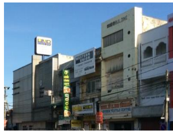
Doors – Commercial shops
