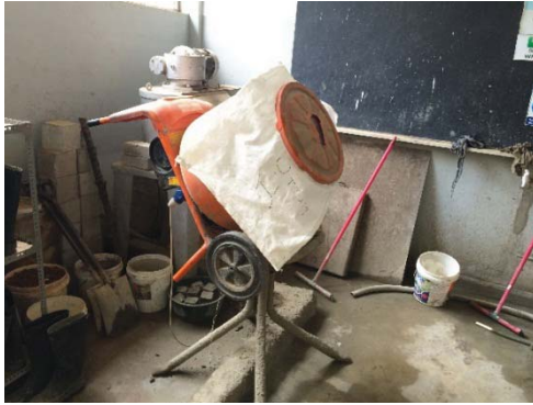
Figure 3.10 Method 1 - Keeping the mix inside the mixer
