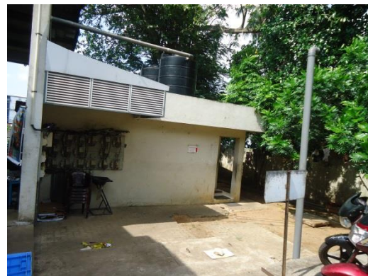
Fig; 12 – public toilets at corner of market [Source: by author]
