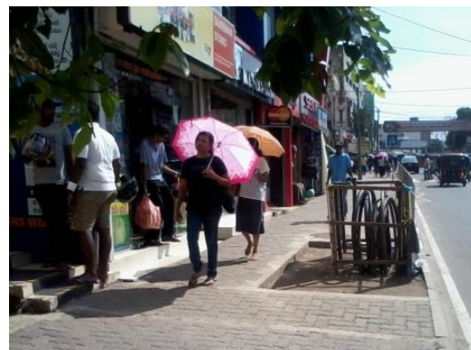
Fig; 42 - Paving were removed for some repairs & they were not replaced again.
