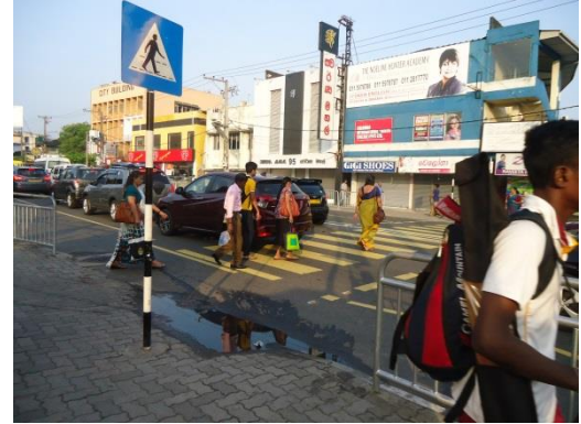
Fig; 31 - pedestrian crossing starting point was filled with rain water in rainy days. [Source: by author]
