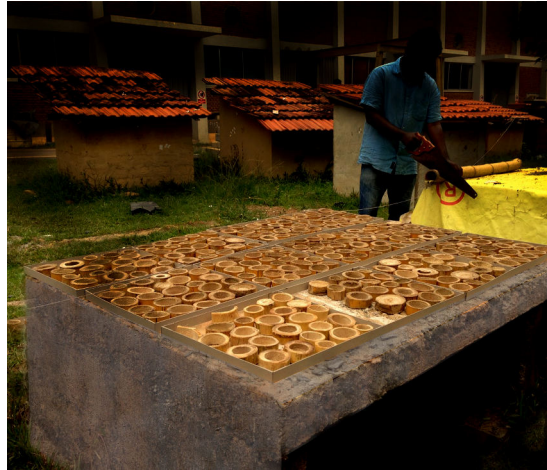
Figure 6.7: Construction of the System with 25mm Bamboo Insulation
