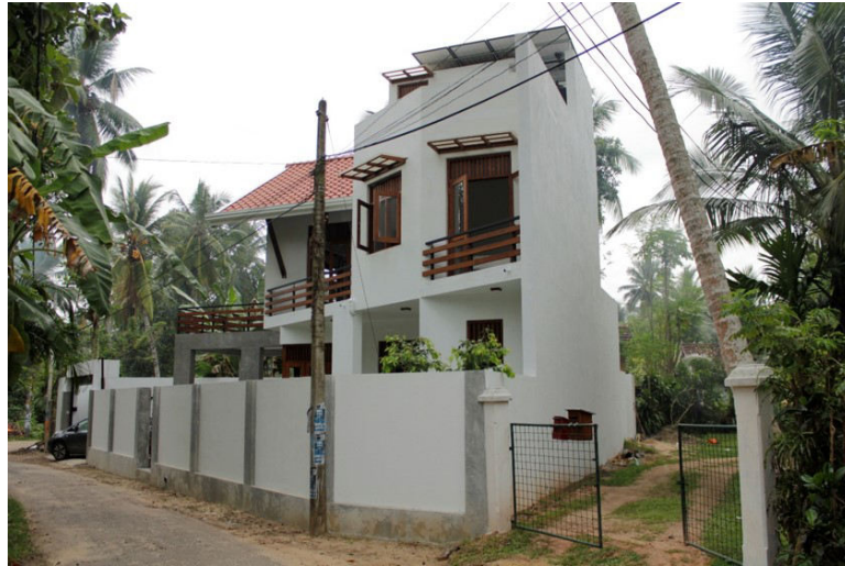
(a) The Building Used to Obtain Thermal Measurements
