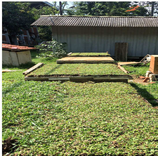
Figure 6.10: Construction of the System with 25mm Bamboo Insulation
