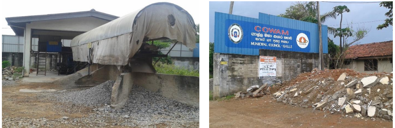
Figure 2 - COWAM Centre, Galle
