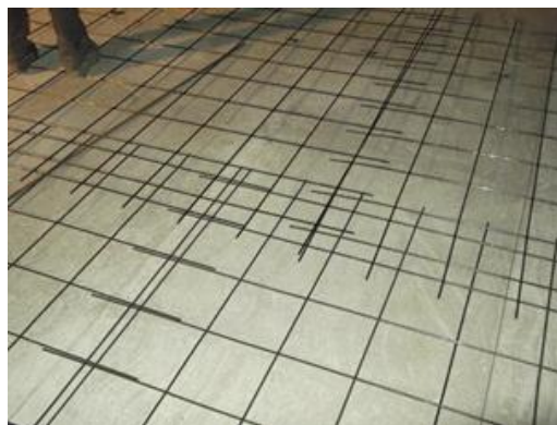
Figure 3.1: Reinforcement net on a pre-stressed slab panel prior to concreting
