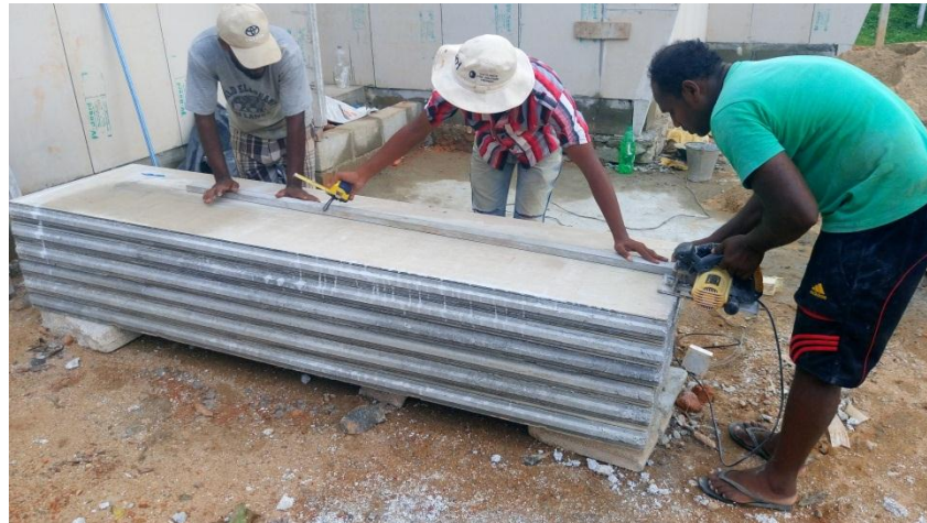
Figure 6.5: Cutting of a wall panel
