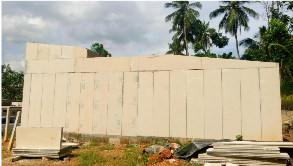
Figure 6.8: Placing of horizontal panels over vertical panels
