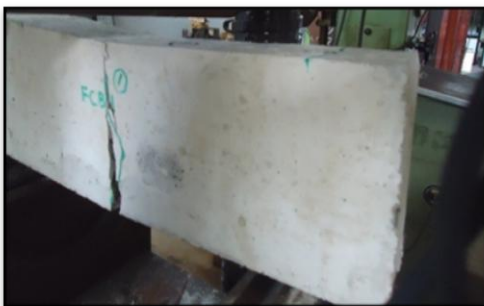
Figure 3.27: Failure pattern of C1
