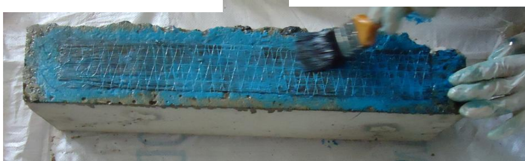
Figure 3.15: Application of saturant on pasted CFRP laminate
