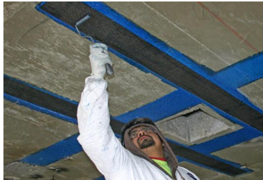
Figure 2.5: Wet layup system
