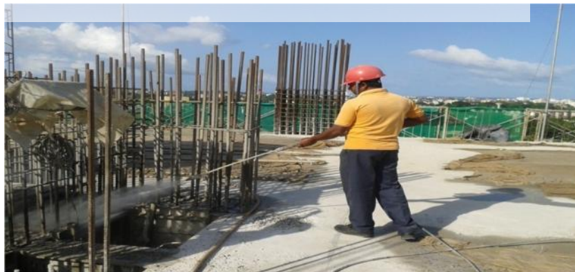
Figure 5.12: High-Pressure Spray Gun Hoses for Curing Concrete Slabs
