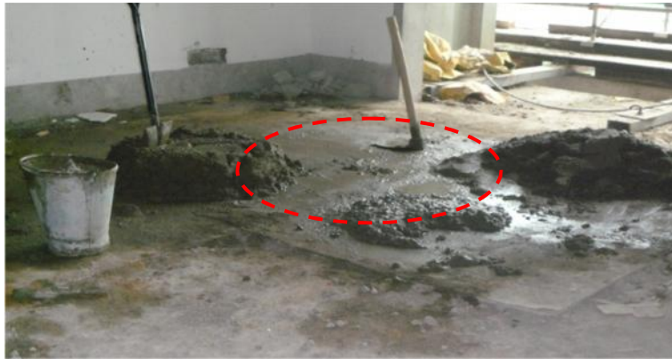
Figure 5.10 : Mixing Mortar on the Floor
