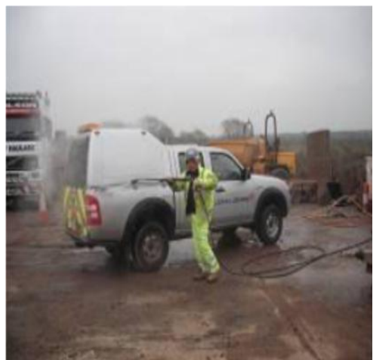
Figure 2.23: Water Efficient Devices: (i) Spray Gun Hoses and (ii) High Pressure Washers
