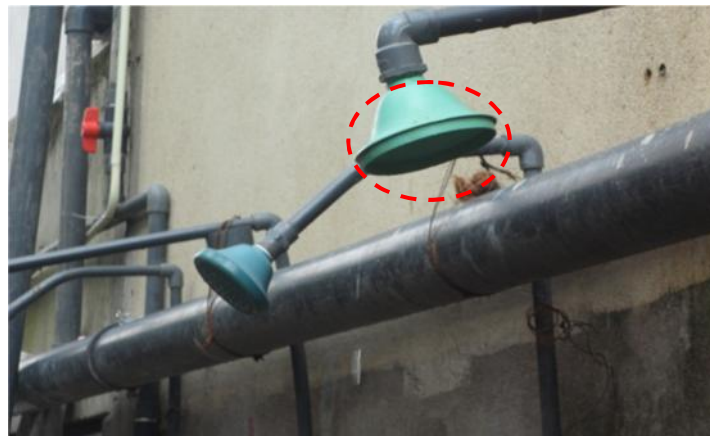
Figure 5.11: Remove Showerheads
