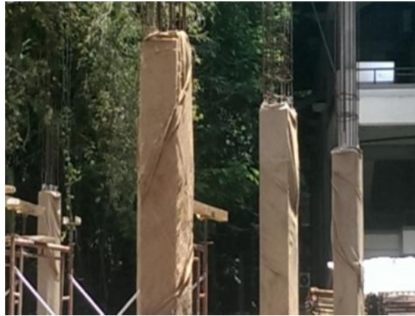
Figure 5.19: Columns Covered with Gunny Bags to Reduce Water Evaporation
