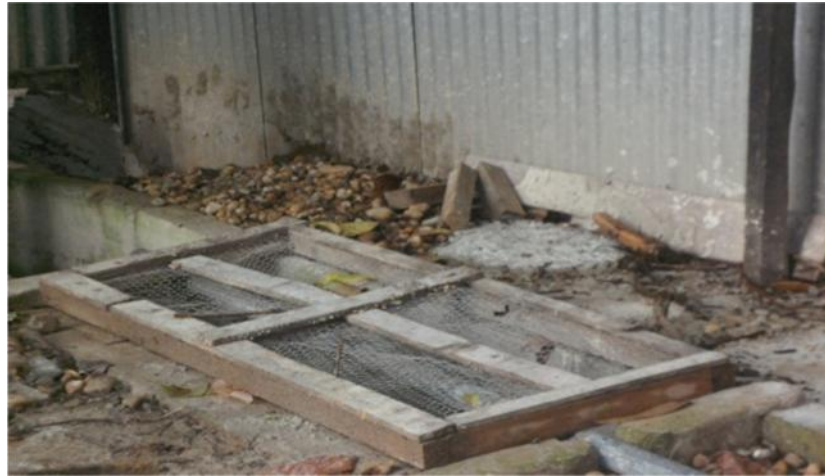
Figure 5.4: The Existing Filtering System Used Prior to Wastewater Disposal
