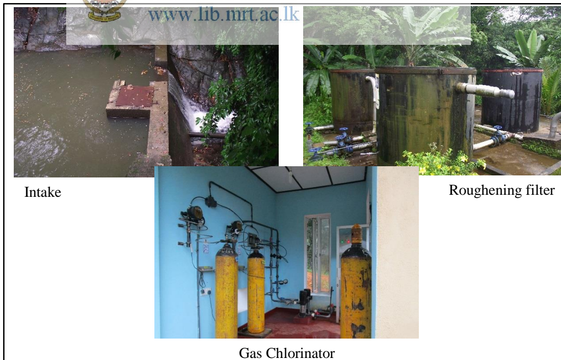
Figure 3.10 – Observations of Eheliyagoda water treatment plant
