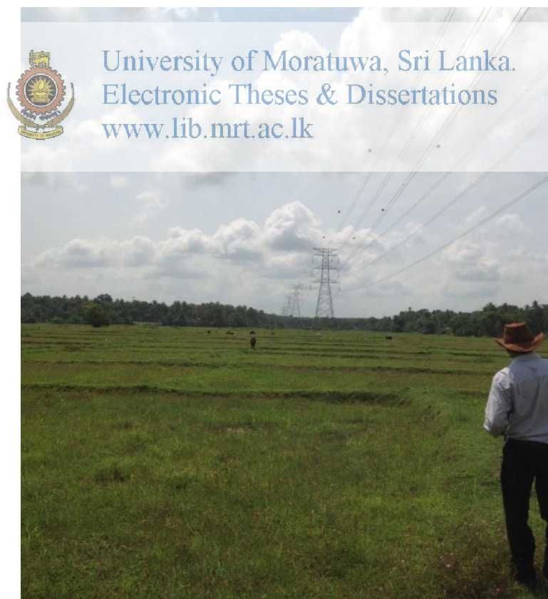
Figure 4.1 Location selected for taking measurements in 220kV line.
