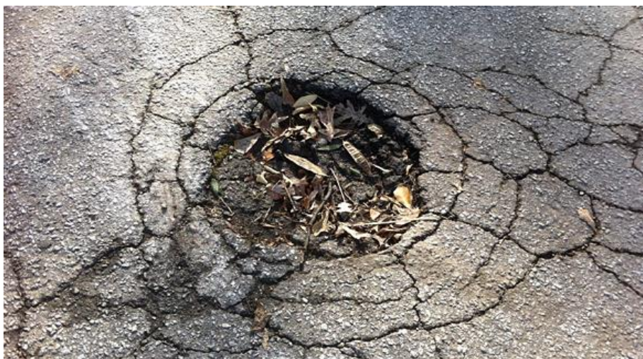
Figure 2-17: Pot holes (original in colour)
