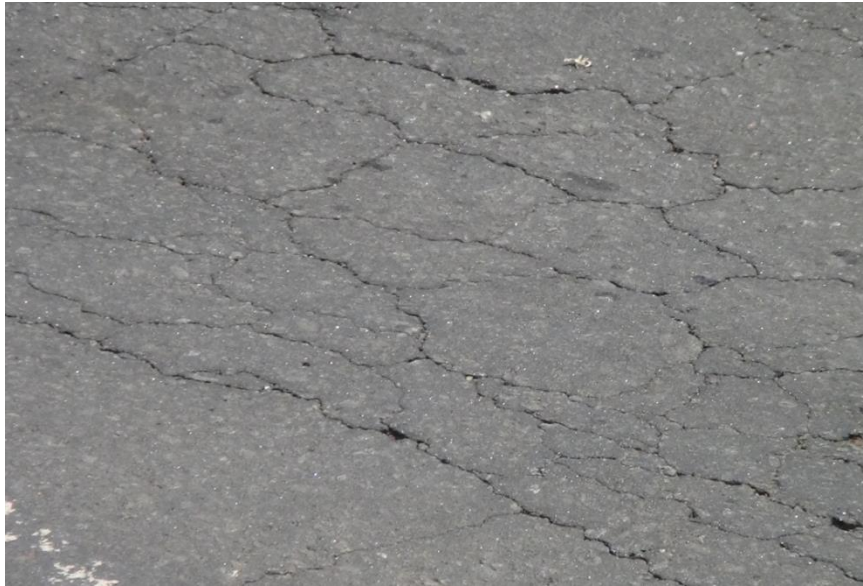
Figure 2-10: Alligator cracking (original in colour)
