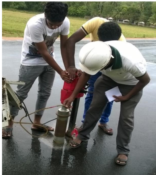
Figure 3-3: Core sample taking before open to traffic (original in colour)
