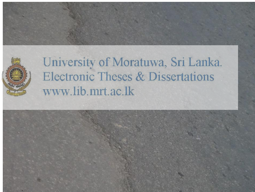
Figure 2-20: Shoving (original in colour)
