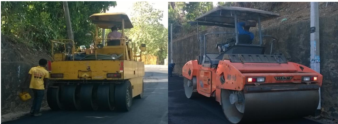
Figure 2-5: HMA compaction (original in colour)
