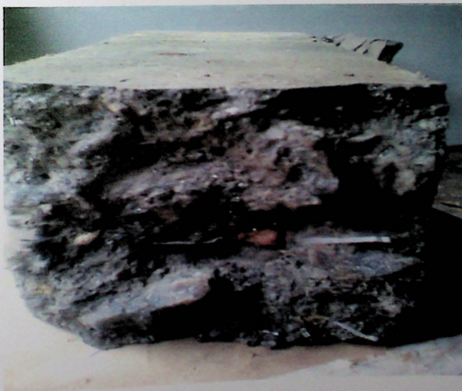
Fig.3.6: The cracked surface of the tested beam
