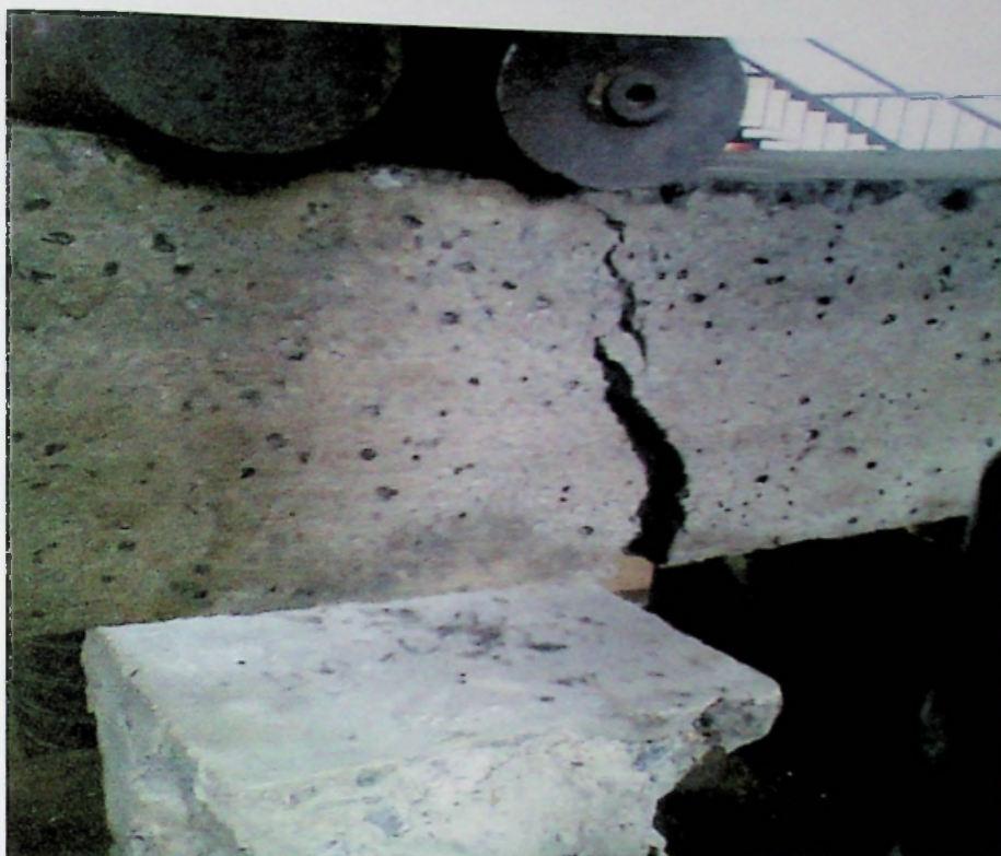
Fig.3.5: The crack was initiated at the bottom and propagated upwards
