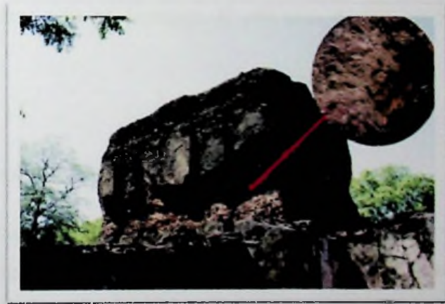
Wind erosion Upper part of the wall in Palace of king Parakramabahu
