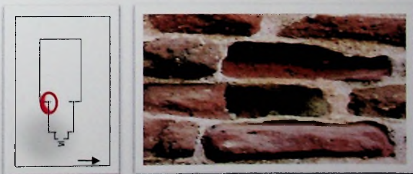
Dissolving bricks in bricks wall
