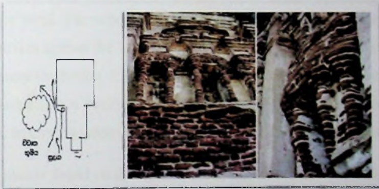
Wind eroded south wall - Thivanka image house
