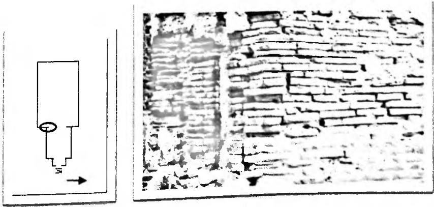
Deterioration of tender bricks and survival of the tough mortars
