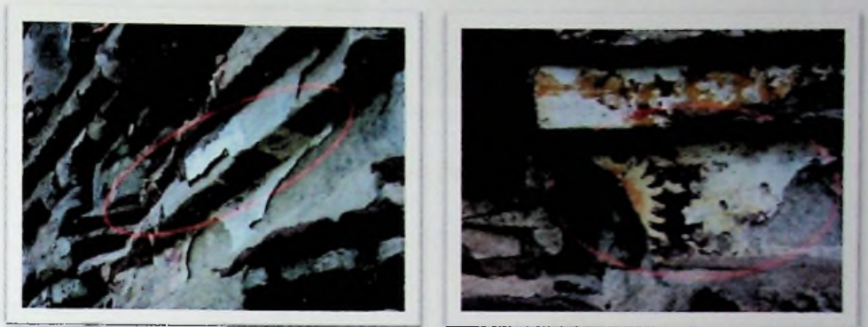
Peeling off so painting and Places where colours are well preserved
