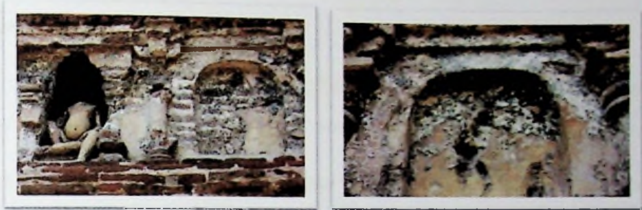
Lichen which grow on the lime plaster
