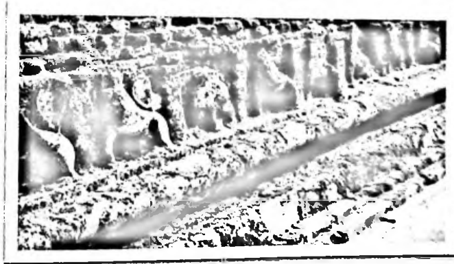
Growth of moss on molding in Lankathilaka image house
