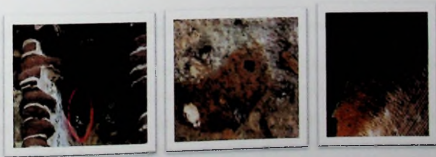
Damage caused by potter-wasps
